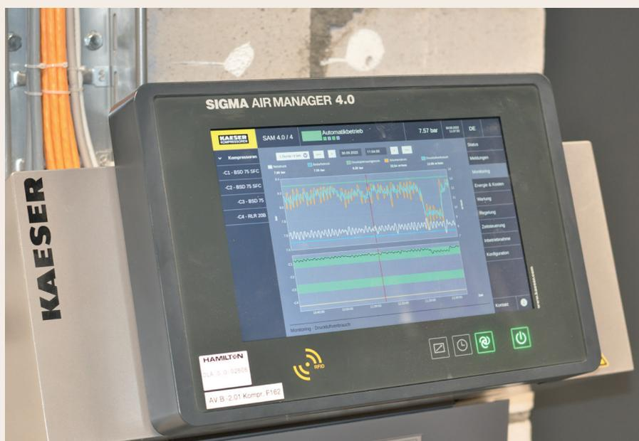
Figure 10: The newly installed compressed air management system, SIGMA 4.0. (Photo: Pascal Kienast)
