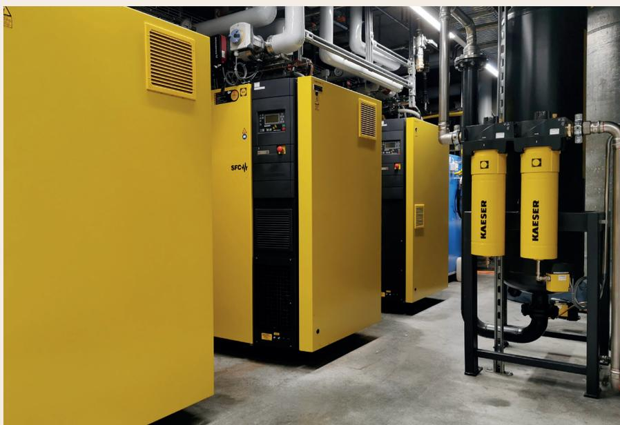
Figure 9: New compressed air system with compressed air management system. (Photo: Pascal Kienast)
