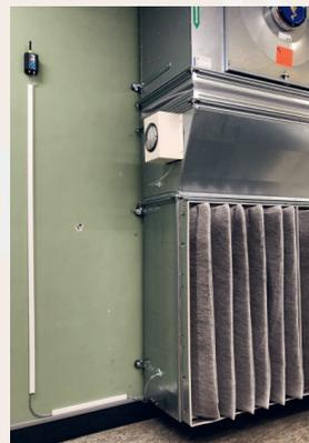
Figure 4: Specific installation of the sensor for the filter system. For the pressure difference, pressure is measured within the ventilation system and in the room (ambient air pressure). (Source: [www.priot.ch](http://www.priot.ch))
