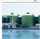
The farm's biogas power generation project uses chicken manure and sewage fermentation to produce biogas. Commissioned in 2009, the facility is powered by three Jenbacher J320 biogas-fueled engines, and a J620 biogas-fueled engine was added in 2018.
