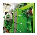
The cogeneration plants installed at BMW Group's' factories in Regensburg and Leipzig can generate on-site power and capture engine waste heat for the factories' production processes. Winter heating is obtained through a combination of the engines' waste heat and heat from existing boilers.
